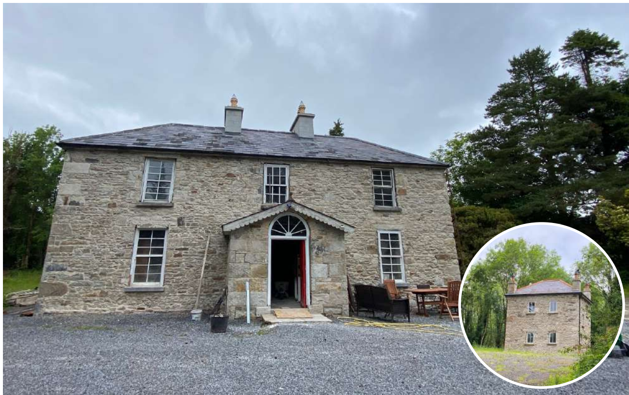
Plate 6: Killedan House is undergoing extensive restoration as is the Tower House (inset) near the entrance gates to the site. The stone walls are devoid of plants at this time. Photos: © C. O'Connell and J. FitzGerald
