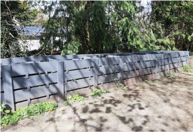
Plate 53: Composting units at the Bog of Allen Nature Centre in Co. Kildare made from recycled plastic lumbar. Each of the bays is filled in turn with a mixture of green and brown organic waste. The provision of 8 bays allows material to compost down over time, facilitates turning and ensures the compost area remains neat and tidy. Action 6.4.12 in Table 7 recommends installation of this type of system in the Crossmolina Community Gardens to compost the shrub and meadow grass cuttings. See https://compostingireland.ie/wp-
