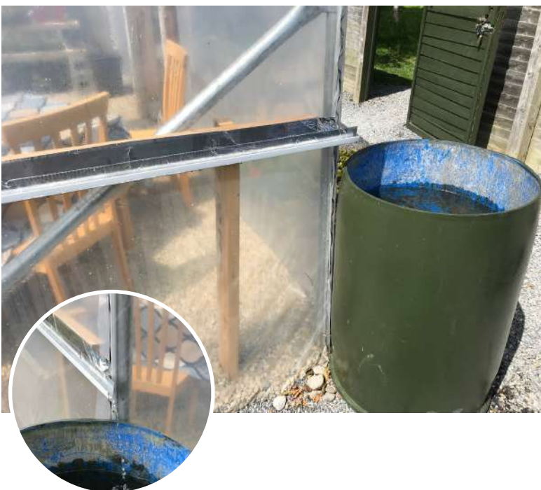
Plate 55: Light weight flexible gutter attached to wooden stakes for collecting rainwater from a polytunnel roof in Ballynahown, Co. Westmeath. This system could be established on the polytunnel in the Crossmolina Community Sensory Gardens and is recommended in Action 6.4.14 in Table 7. Photos: © C. O'Connell
