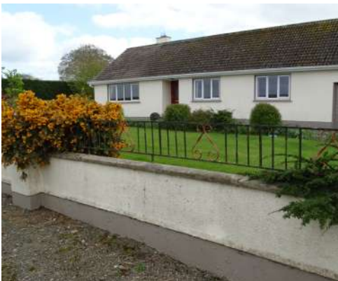
Plate 36: A modern wall habitat outside a home on the L8006/7 showing the lack of wildlife colonisation. Action 8.6.9 in Table 10 provides suggestions on screening plants that will enhance biodiversity. Photo: © C. O'Connell.
