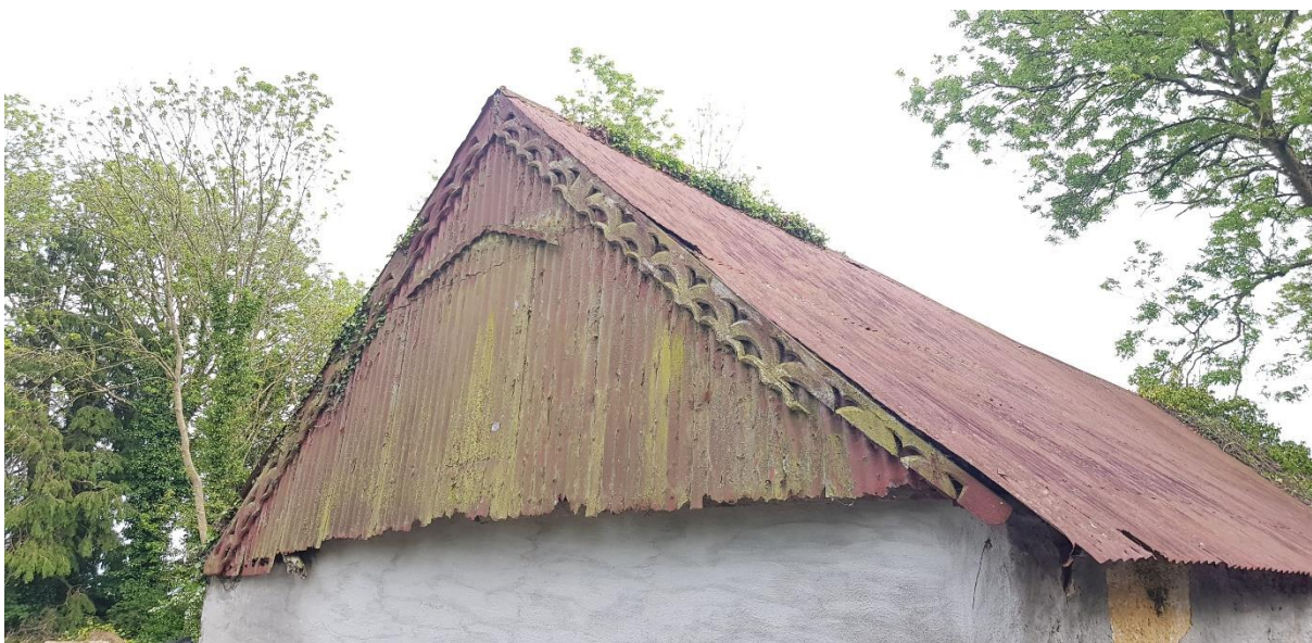
FIGURE 7 VERNACULAR HOUSE AT CLARSON'S CROSSROAD WITH UNIQUELY CARVED FASCIA
