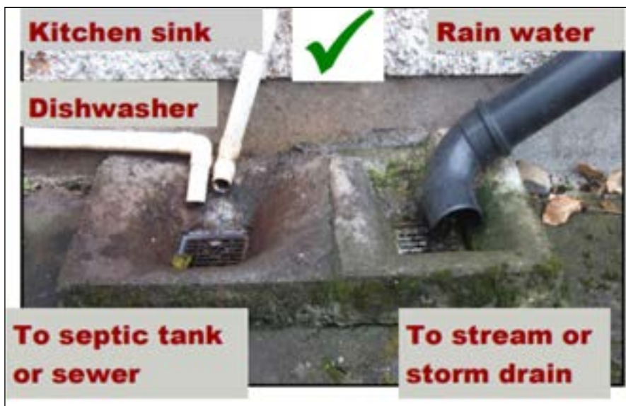
Figure 36. Correctly plumbed premises.
