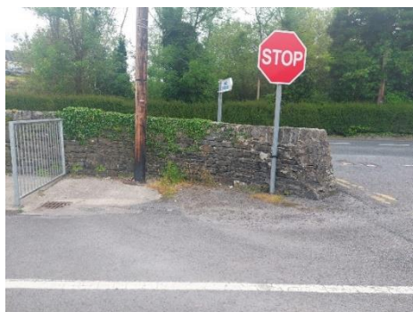
Area of carpark (marked B on map) where a planter could be placed.
