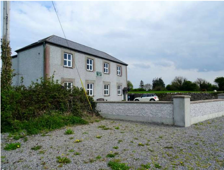
Figure 12: The community centre in Tang is located in the old school building. This building is recently refurbished and has little biodiversity value. In the gravel area shown above, a Wildflower welcome area is suggested to enhance wildlife (see Action 8.4.1 in Table 8.4) and Figure 13. Photo: © C. O'Connell.
