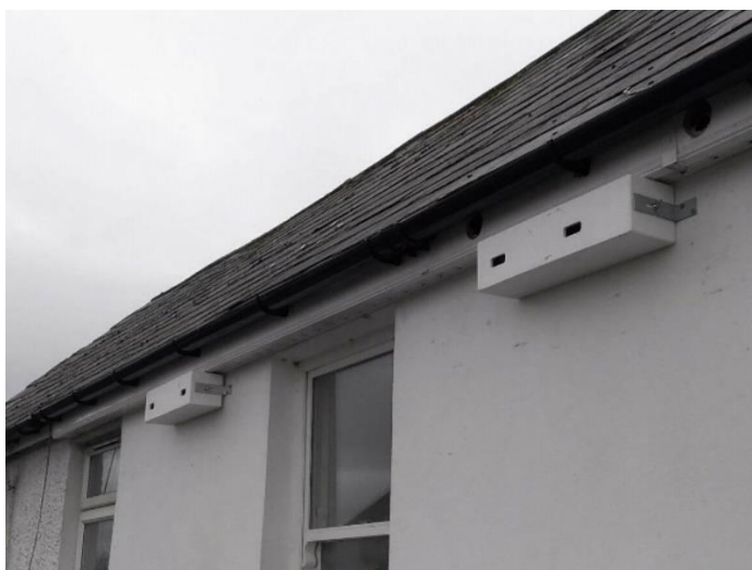
Plate 28: External Swift boxes at Tralee, Co. Kerry – Copyright © Anthony Dawson. Source: Swift Conservation Ireland
