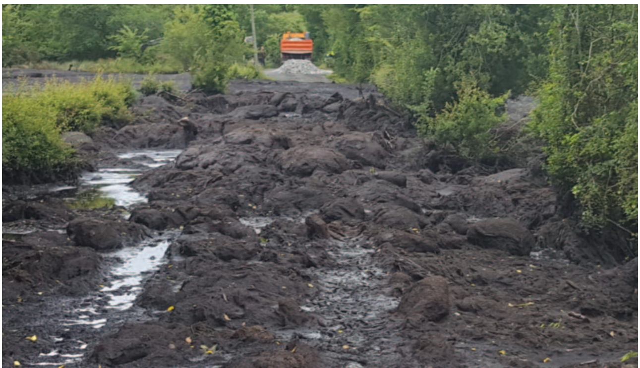
Figure 35: Bog slide at Drumkeeran from Shass Mountain, Co. Leitrim. The bog burst due to works associated with a wind farm construction in 2020. Photo: © T. Moseley
