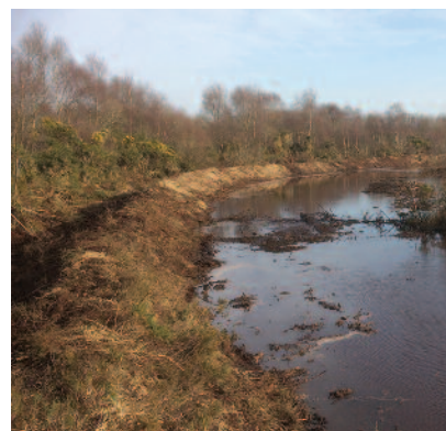
Figure 24: Barrier dam constructed on Ardagullion Bog in 2019 as part of the Living Bog Restoration Project to provide peat-forming conditions in the cutover bog. Photo: © J. McGawley
