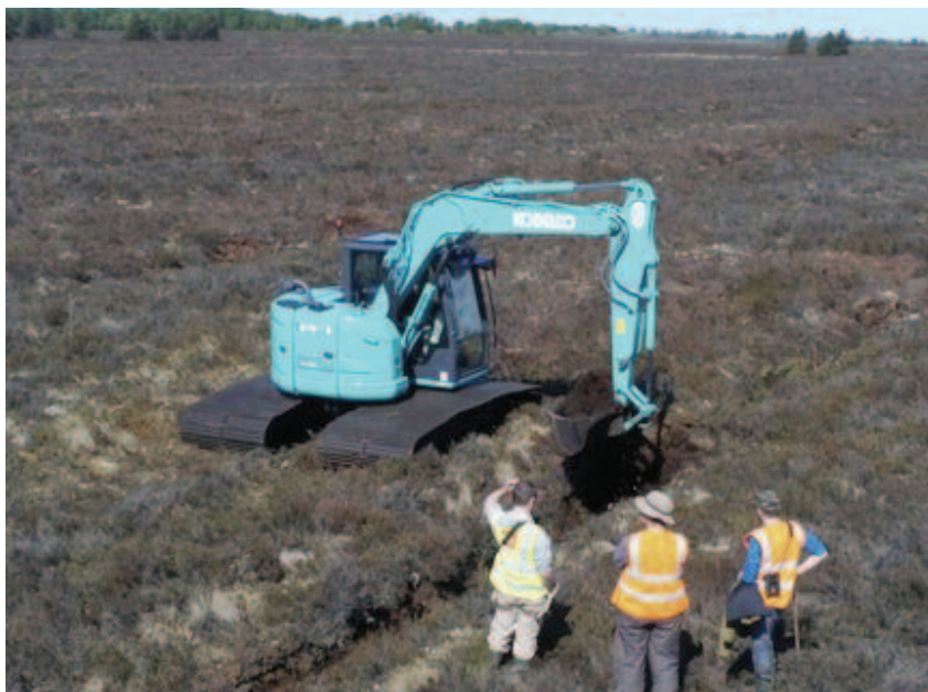
Figure 22: Specially adapted machine developed by Bord na Móna to construct peat dams on bogs of conservation importance. Photo: © Bord na Móna
