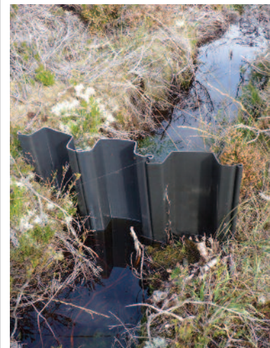
Figure 23: Drain with high water table after blocking with plastic sheet piling on Lodge Bog, Co. Kildare in 2010. Photo: © M. Kenny
