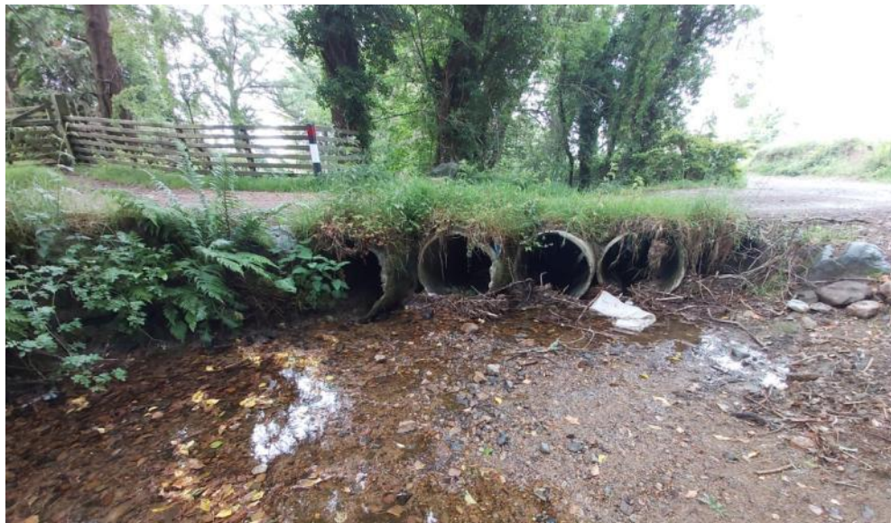
These pipes together with the step drop downstream present a significant obstacle for fish and other aquatic species
