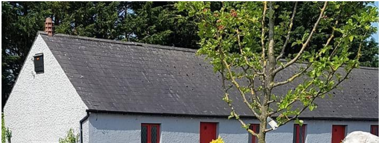
Figure 9 – Bat Box Located on Gable Wall of Old Hall
