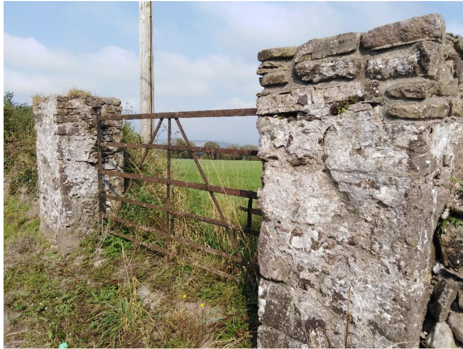
Fig. 10 Traditional gate and gate posts almost opposite the former Shamrock pub
