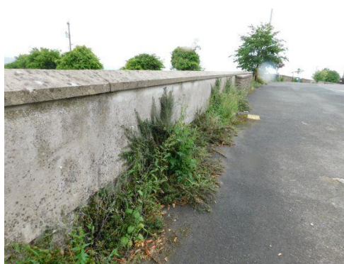
Image 14. Church car park
