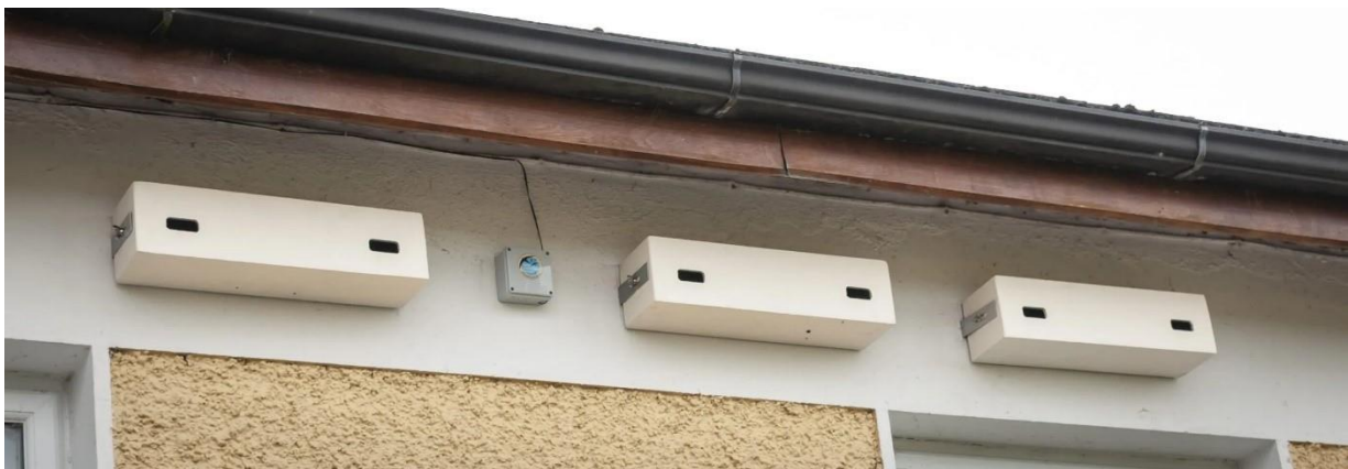
FIGURE 17. SWIFT BOXES UNDER EAVES.
