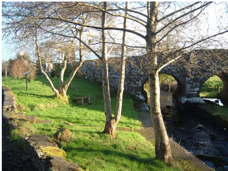
Bridge over Derryhippo River
