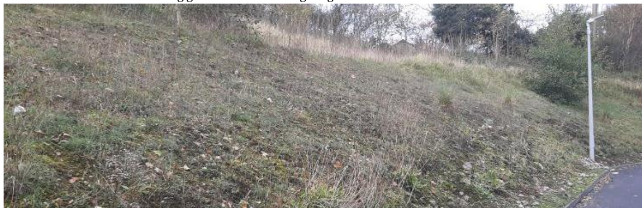
Plate 13: Bank of re-colonising ground at Circle K garage
