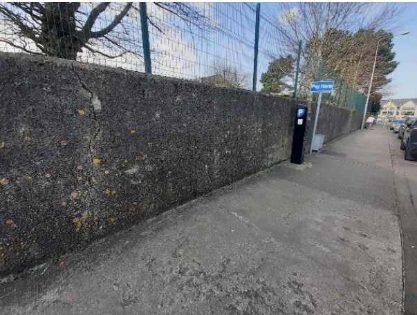
Plate 10: Bare wall outside of the school, potential site for mural
