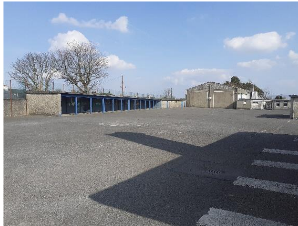
Plate 11: Bare area of concrete/ tarmac yard beside the school.
