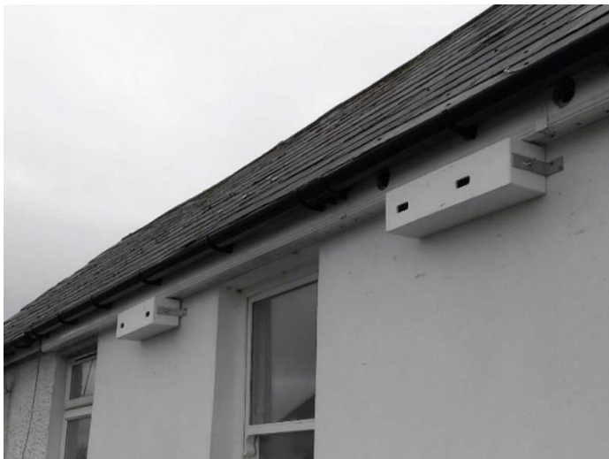
Plate 1: External Swift boxes at Tralee, Co. Kerry – Copyright © Anthony Dawson. Source: Swift Conservation Ireland
